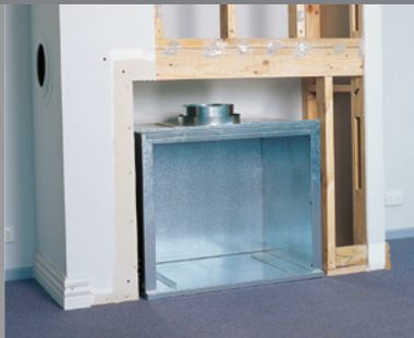
Zero Clearance Box positioned in framework on 18mm sheet
